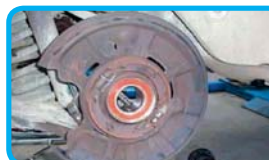
HUB INSTALLATION FINISHED
